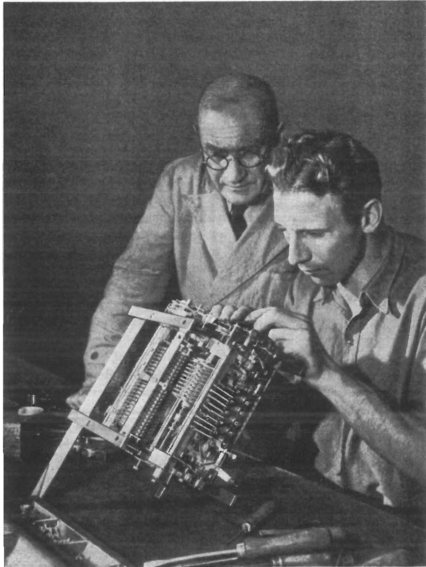
Constructing a "Facit" calculating machine, perhaps the most famous of the many well known office machines made by Åtvidaberg. Photo: Åtvidaberg.
